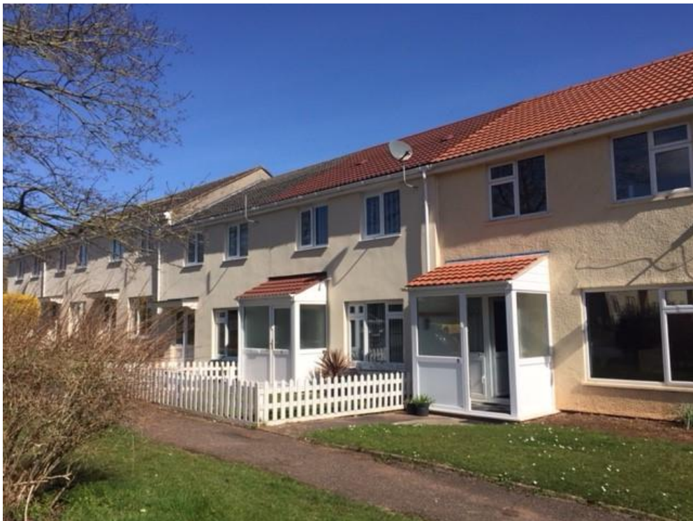
Fig 2. Contrasting completed properties adjacent to private homes
